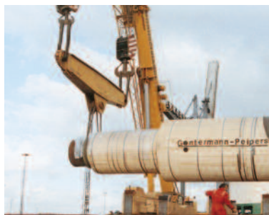
Transfer from rail to skid/cargo bridge combination by 4 mobile cranes.
